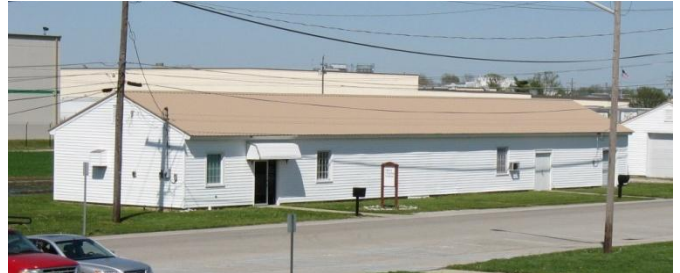
Here's what one of the five buildings (Liberty Christian Academy) looks like with its new tan metal roof. All 5 buildings look like this one.
